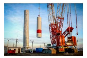
Before lifting, each section of the tower is removed from the car trailer and cantilevered (translated into a vertical position) using two cranes. Then it is lifted and installed in the design position (height - 15-22 m, weight - 56-61 tons).
