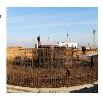
concrete preparation - pouring a monolithic slab with a diameter of 18 meters and a thickness of 260
