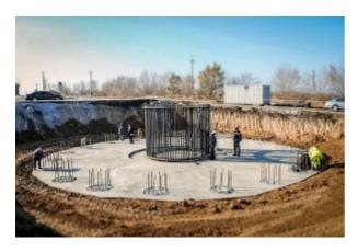
mm, on which the reinforcing frame is installed. Special parts (retainers) for mounting and checking the anchor device are also laid in the concrete preparation. A distinctive feature of foundations for WPPs is the extremely high saturation of steel reinforcement. The step of reinforcement in the frame does not exceed 100 mm, which required the use of vibrators when laying concrete. Concreting of the foundations was carried out
